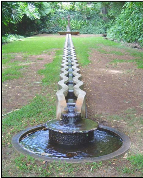
The original and clever irrigation system at Allerton Garden (Photo 3).
