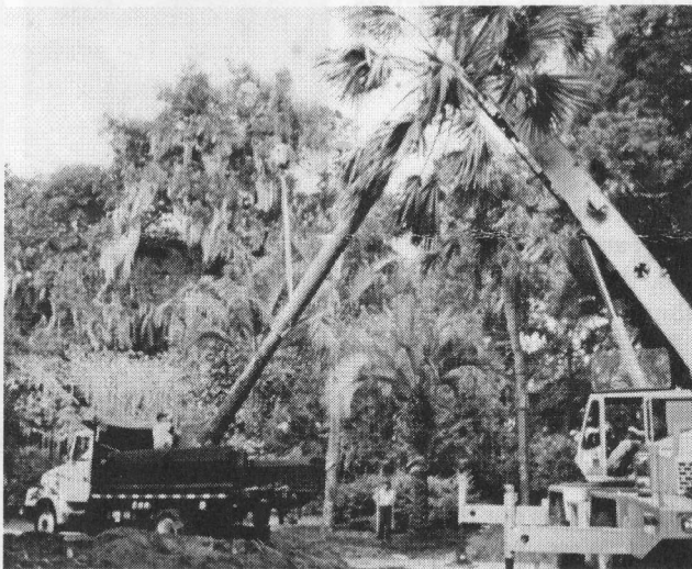
Figure 1: A massive Sabal causiarum weighing 7,600 lbs. is hoisted by a crane into an awaiting truck.
